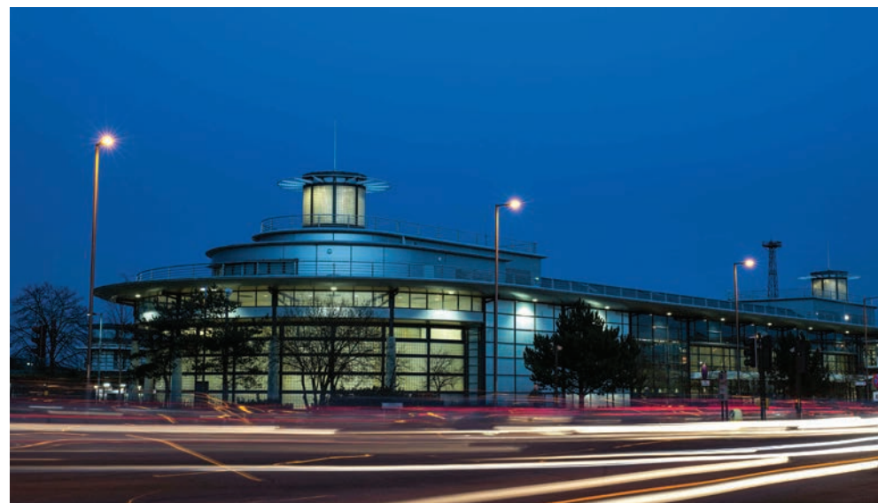
Ashford International Railway Station
