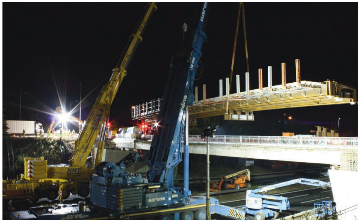
M20 Junction 4 overbridge widening
